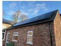
Solar Panels on Allerthorpe Village Hall, funded in 2024
